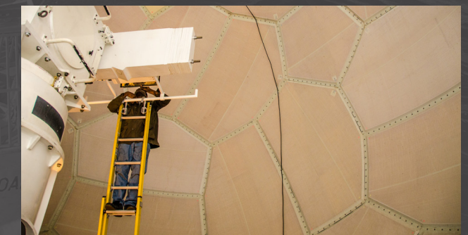
Maintenance being performed at the Chicago NEXRAD located in Romeoville, IL.
